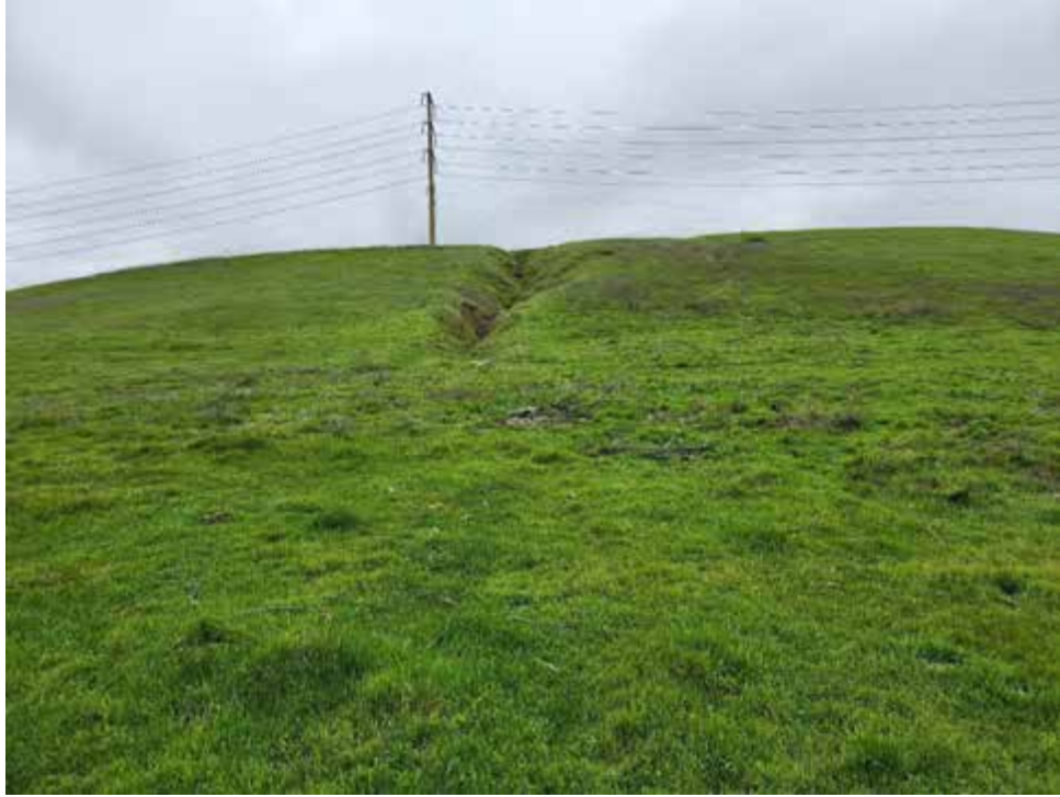
View looking west of a graded commercial pad with an erosion gully in a pasture setting
