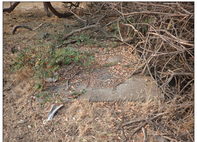
PHOTO 4: Water Main Covers
