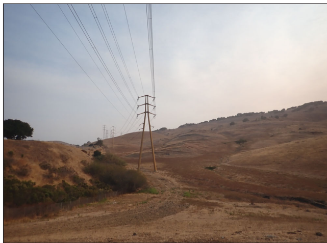
PHOTO 3: Western Power Line.
